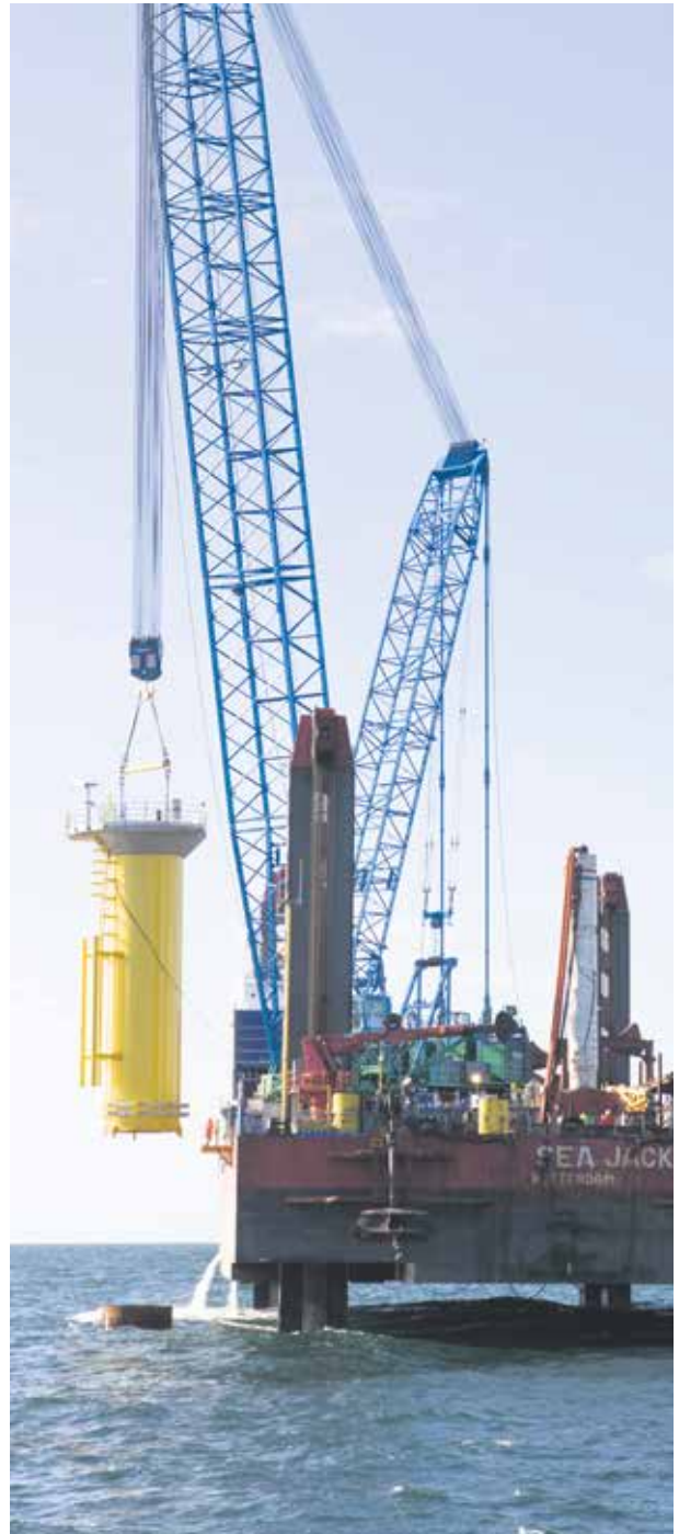
Construction of monopile foundations at Horns Rev 2.
